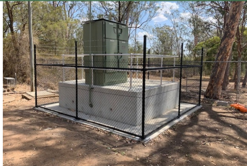
Chainwire around a pump station
