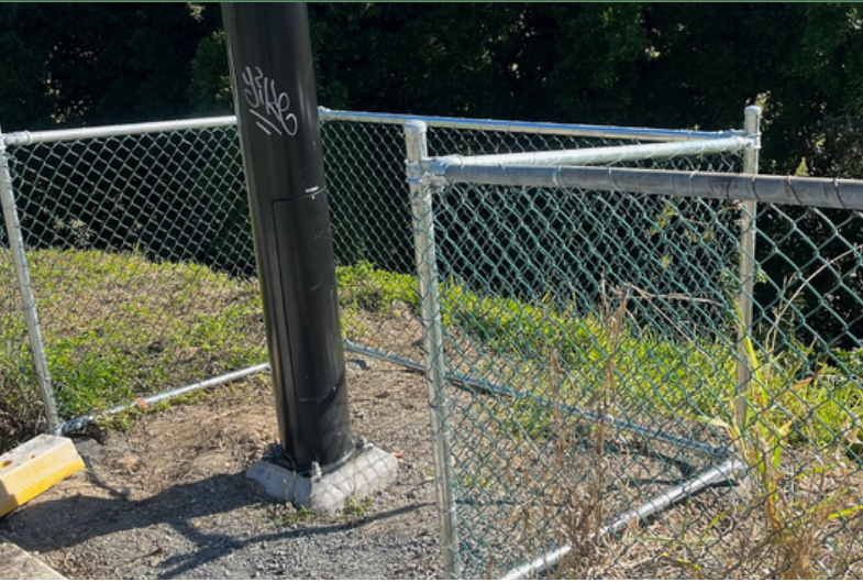
1200mm high fencing around light posts on a walkway
