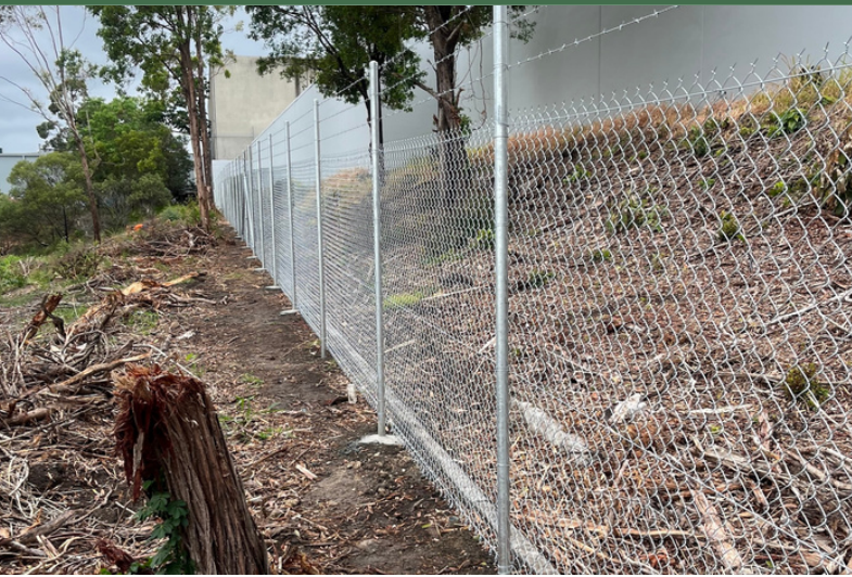
1800mm high chainwire plus 3 rows of barbed wire
