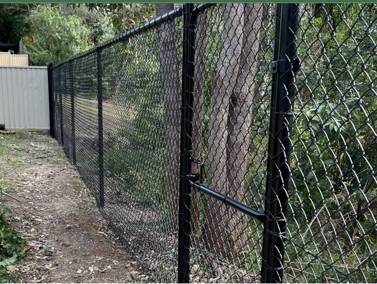
1800mm high fencing with a single gate and horizontal rail
