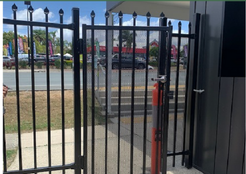
Single 1800mm high security gate with mesh
