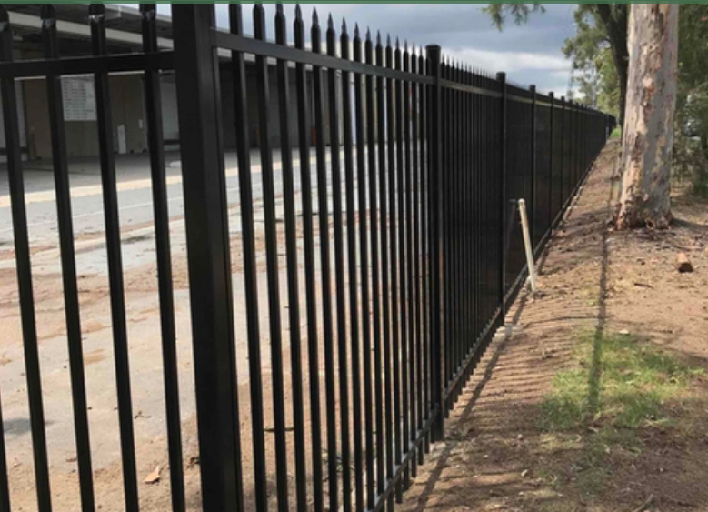
2100mm high steel security fencing for a High School
