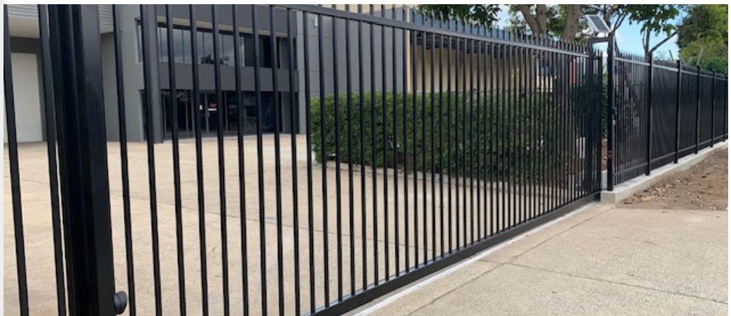
9 metre sliding gate
