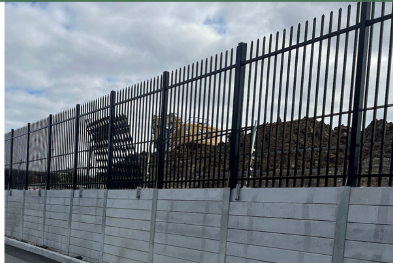
DETE Spec Fencing on a Retaining Wall
