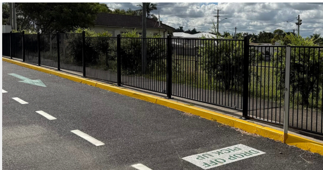
1200mm high Aluminium Fencing for a drop off zone
