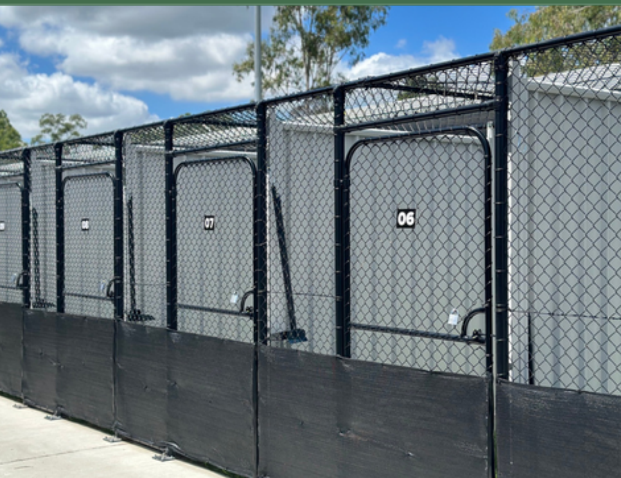
Chainwire dog enclosures with chainwire roof and 2100mm high colorbond dividers with posts set into block wall.
