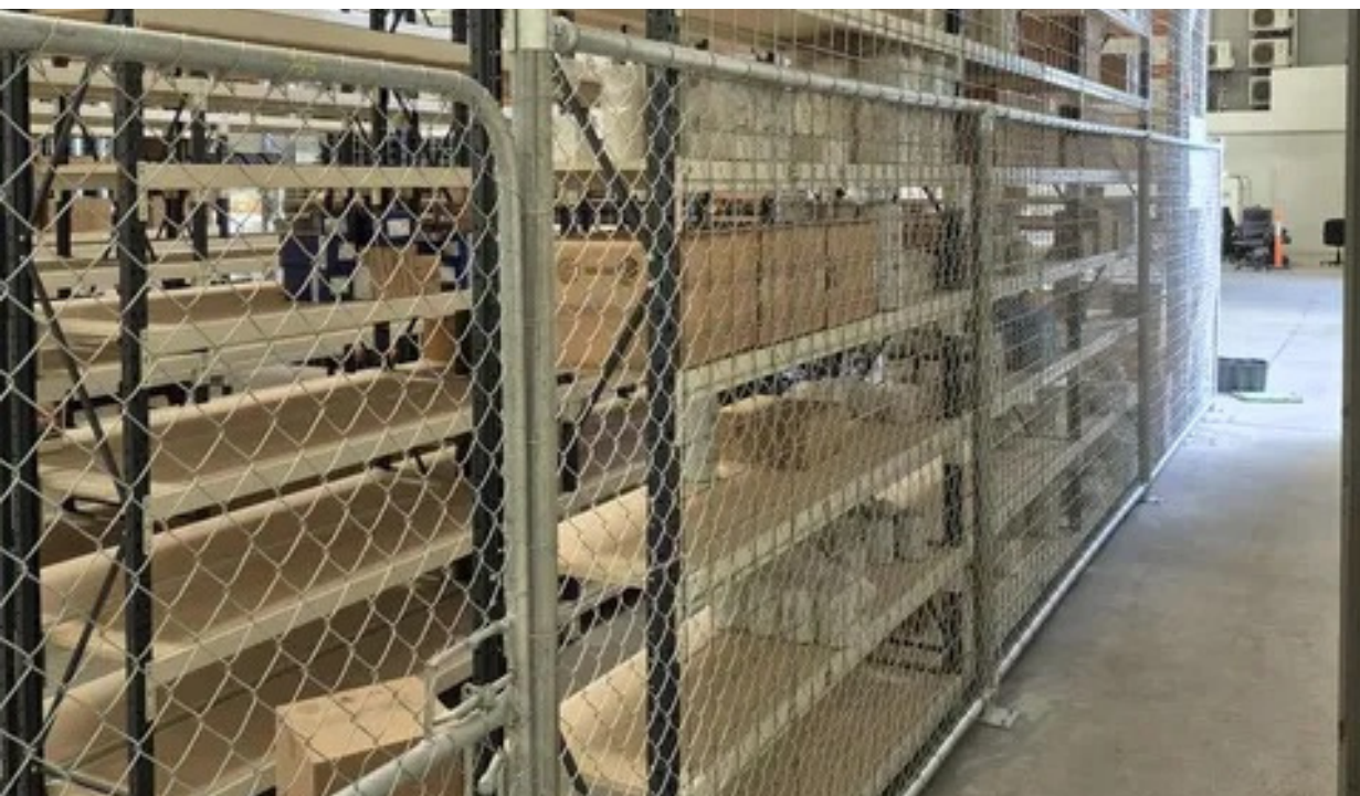
Chainwire fencing in a warehouse
